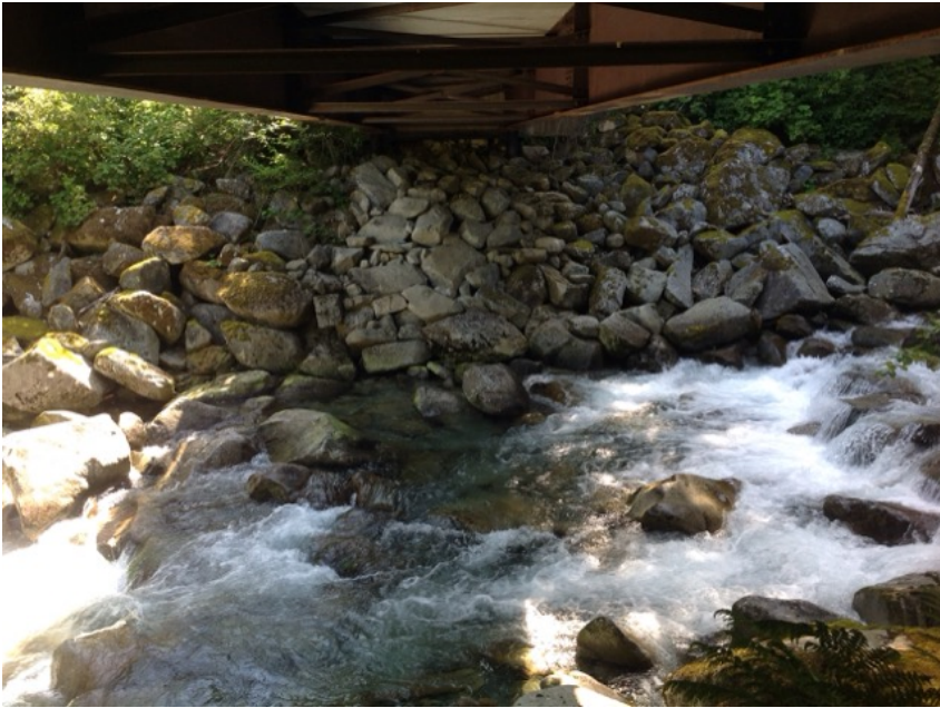
Right Bank Abutment when facing downstream
